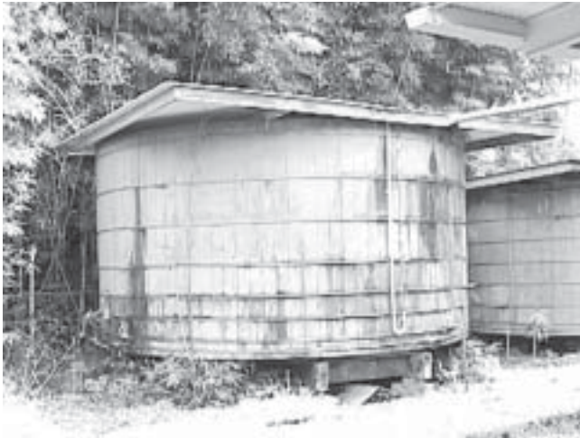
An older redwood tank. Beware of redwood tanks that were painted on the inside with lead paint to discourage algae.
