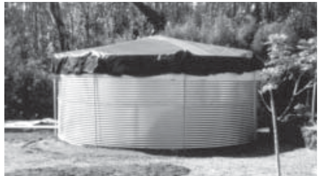
Pipe arches supporting a mesh cover keep it from sagging into the water.
