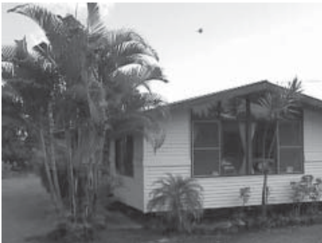
Do not allow trees and bushes to overhang your roof. They provide roof access to rats and other vermin.
