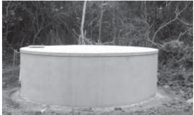
Ferroconcrete tanks, also known as ferrocement tanks, are new to the local market and growing in popularity. Like solid concrete tanks, they can be designed into a home's structure.
