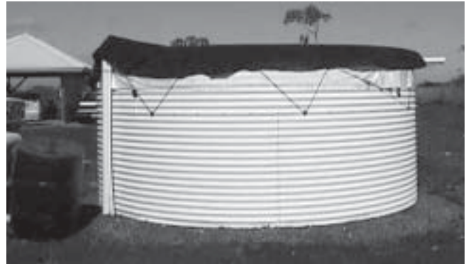
A typical corrugated steel tank with a mesh cover. This type of tank is the second most common in use today.
