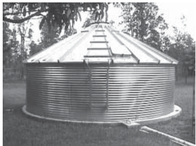
Some galvanized tanks have solid covers. This model has a top hatch for access and a liner secured to the sides with bolts.
