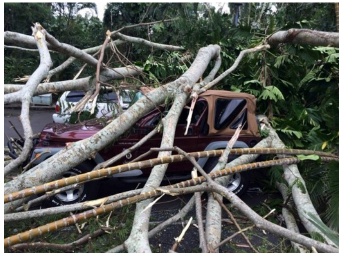
Figure 3: Property damage caused by fallen albizia branches. Photo provided courtesy of BIISC.
